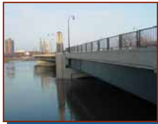
Main Ave. Bridge
